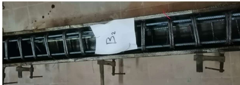
FIGURE 2. Wooden form and reinforcement of the concrete beams
